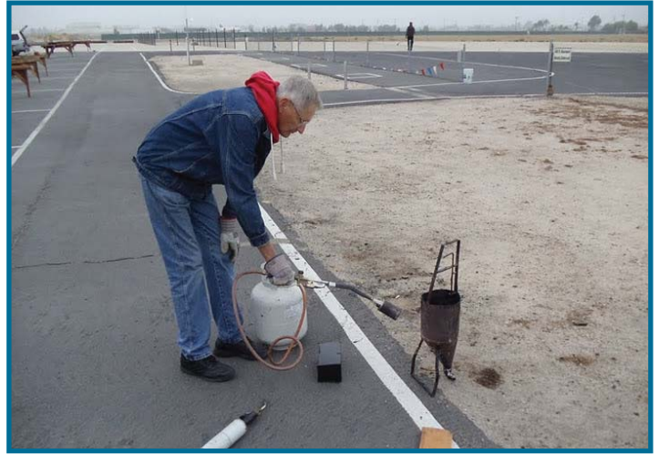
Paul Smith warming up the tar to flow into the cracks.
