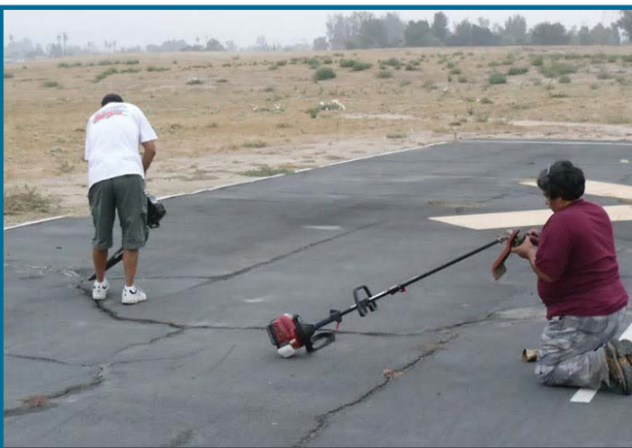
Removing the weeds out of the cracks.
