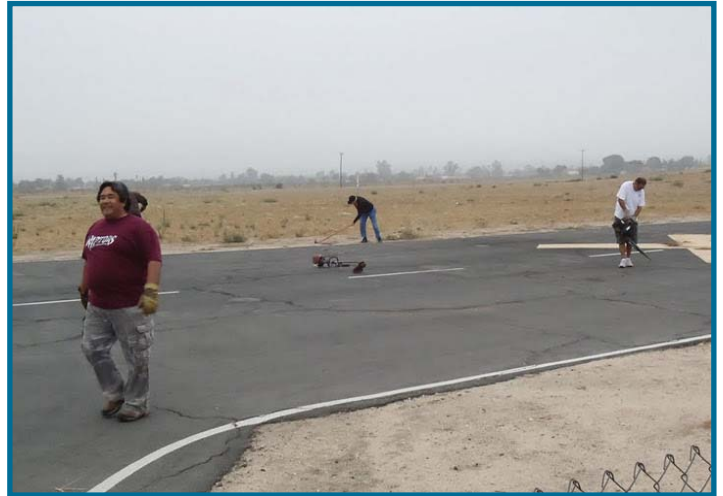
Everyone was busy filling cracks.
