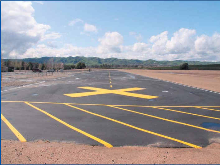
Approach to the PVMAC Prado Airpark Field...just after surfacing and new stripping. 800' X 50" Note the small spec midway on left...that is Sam Wright at Pilot Box
