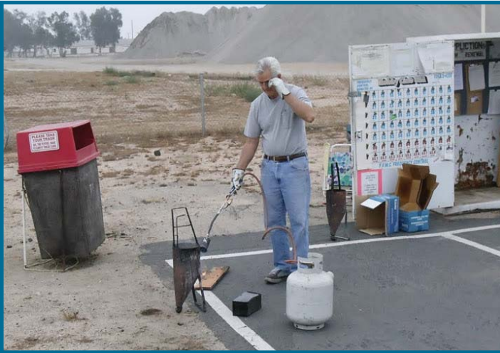
Special Tar Filling Funnels were used on cracks.
